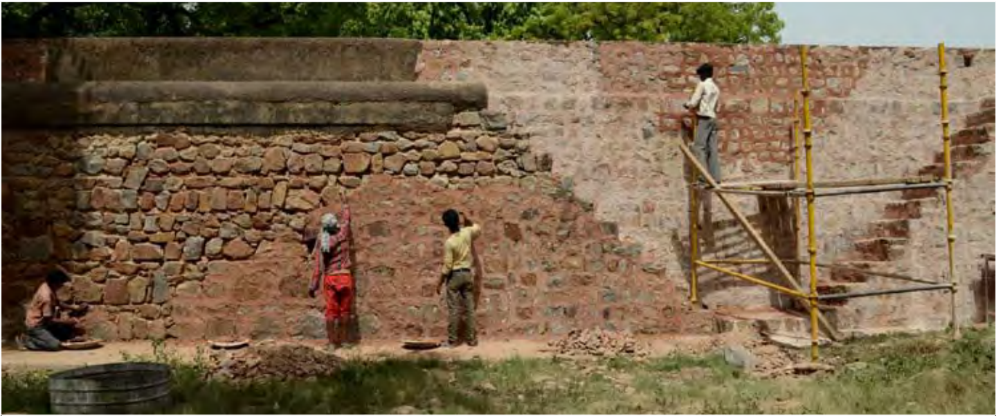
(Above) Removal of dead cement pointing and stitching the cracks in the enclosure wall and bastion chambers was followed by pointing with lime mortar.
