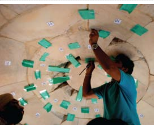
(Top) 19 th century archival painting of Chausath Khamba; (Middle) A detailed architectural documentation of the structure, and (Bottom) stone-by-stone assessment of the structure showing cracks and condition of the domes prior to commencement of conservation works in 2011
