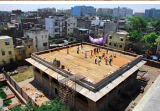
The manner in which this complicated conservation work was undertaken bears remarkable tributes to Indian master craftsmen. (Top) Stitching and grouting of cracks in the masonry while dismantling marble blocks for repair; (Middle) Cracks on the terrace were allowing water penetration and resulting damage; (Bottom) repairs on the roof by adding a layer of lime concrete with traditional additives like Jaggery and Bael fruit pulp.
