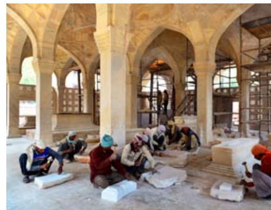
(Above) Various stages of conservation of one dome: 1. Numbering each stone; 2. Dismantling the marble blocks and repairing of cracks in the masonry; and 3. Repair of marble blocks with indents of matching stone where these had burst by master craftsmen using tools, techniques used by the original builders and 4. Re-installation of marble blocks in the original location.
