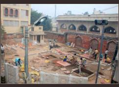
The iron fencing of Mirza Ghalib's tomb enclosure is being replaced with a stone masonry wall with sandstone lattice screens that will help create a courtyard effect and also lend considerable historic character to the principal street leading to the Dargah
