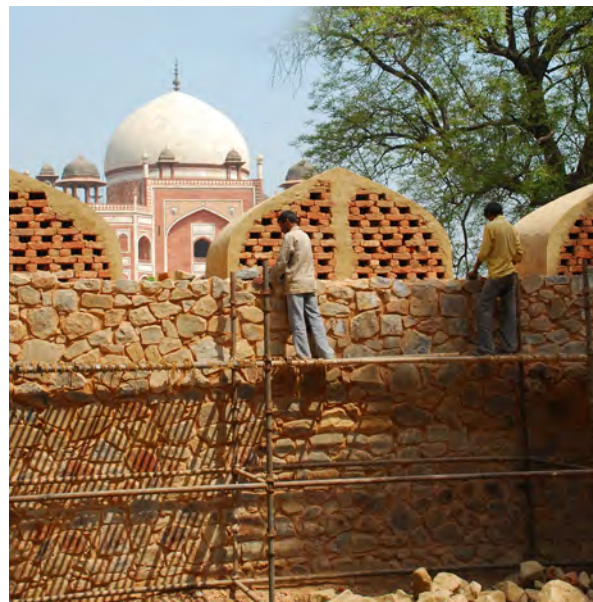
Stone carvers (top), plasterers (central) and masons (bottom picture) used traditional materials building techniques and tools to restore the intention of the Mughal builders
