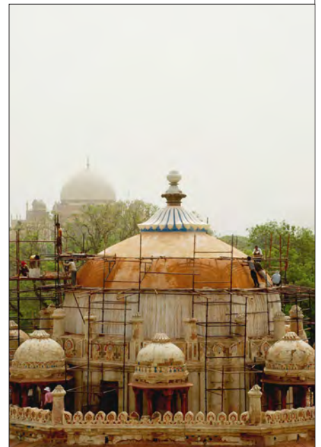
▲ Conservation works on the tomb have included major structural repairs on the dome, restoration of the ceiling and the finial. Restoration of the tilework will carry on through 2013
