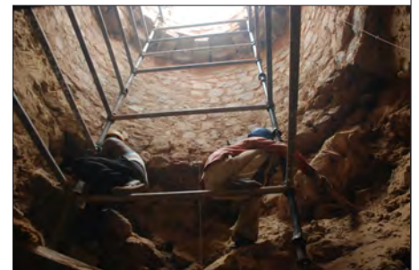
▲ De-silting of historic wells in the project area, and removing decades of rubble and deposits from them
