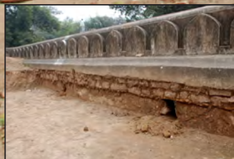
Earth removal led to the arched openings of the outer enclosure wall being revealed to their full height and extent
