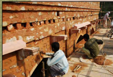
Following structural repairs to the domed ceiling, the battlemented parapet wall was re-built using traditional materials, tools and building techniques
