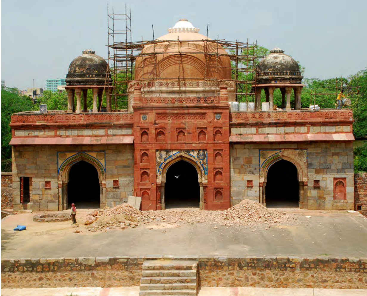
Remnants of tilework on the façade and the canopies
