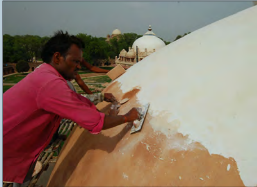
Lime punning being applied to the dome surface
