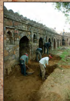
Earth removal led to the arched openings of the outer enclosure wall being revealed to their full height and extent
