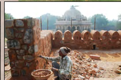
Following structural repairs to the domed ceiling, the battlemented parapet wall was re-built using traditional materials, tools and building techniques
