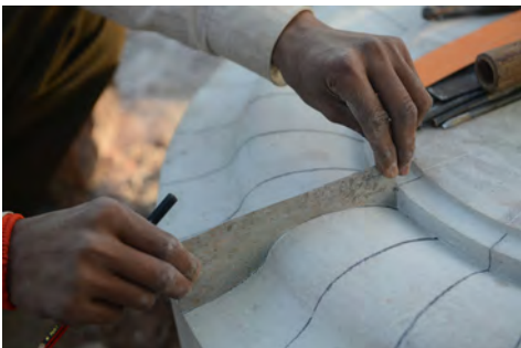
Broken portions of the finial were found collapsed on the roof. Master craftsmen prepared matching finial pieces to restore on the dome.
