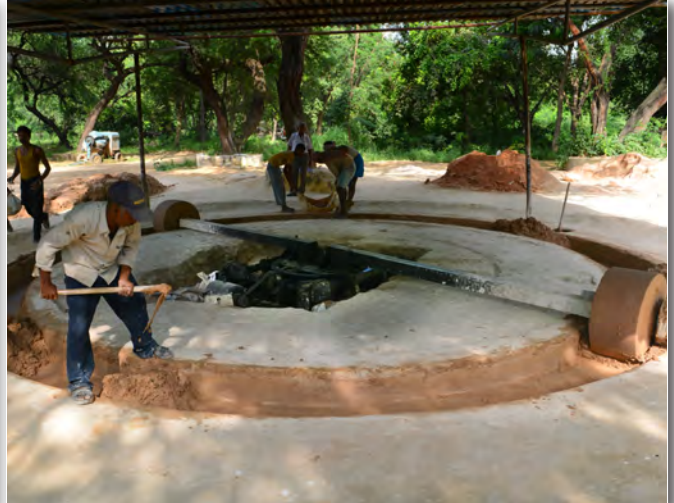
Reviving traditional building craft of Lime
