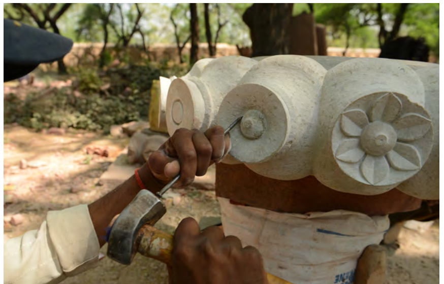
Broken portions of the finial were found collapsed on the roof. Master craftsmen prepared matching finial pieces to restore on the dome.
