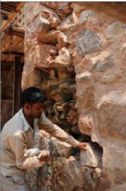
(Left) Consolidation of the collapsed portions and (Below) View of South facade of Mirza Muzaffar Hussain's Tomb during conservation
