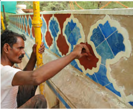
(Above) Tiles, where missing, on the parapet were restored as per the original design and specifications
