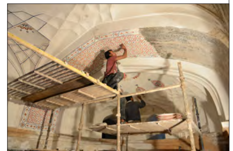
▲ Reconstruction of the missing incised plaster pattern on the dome ceiling, arch soffits and internal wall surfaces
