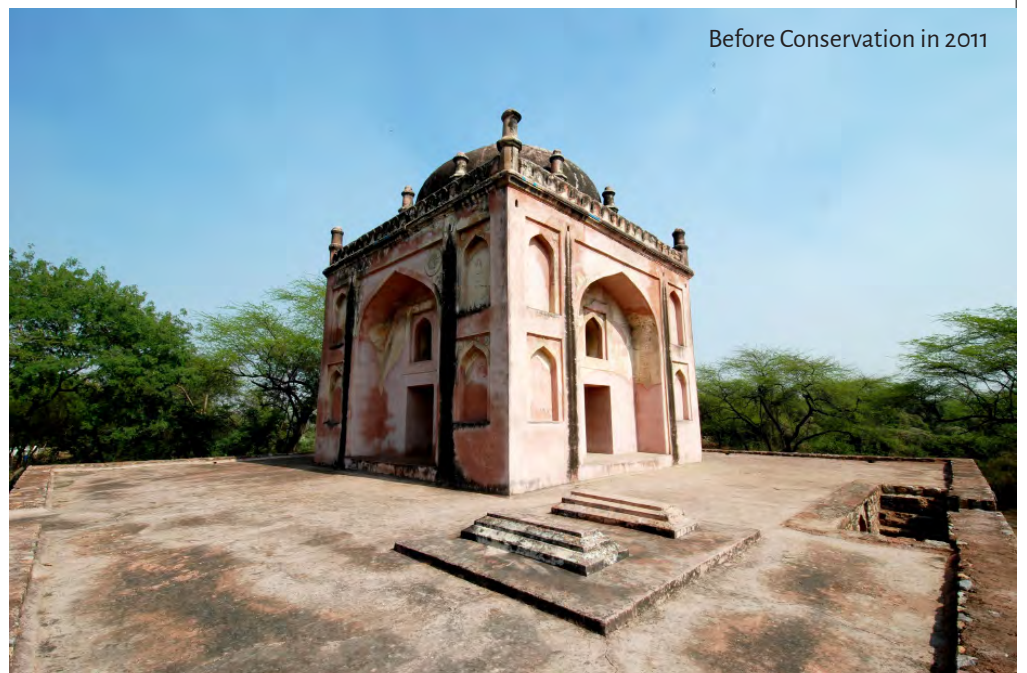
At the Mughal Tomb, a sandstone plinth replaced the earlier cement plinth (Below) which was found to have been laid over construction rubble. The sandstone is long lasting, especially in view of the large number of visitors expected to visit here in future years.
