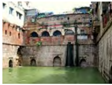
Baoli wall collapsed in July 2008
