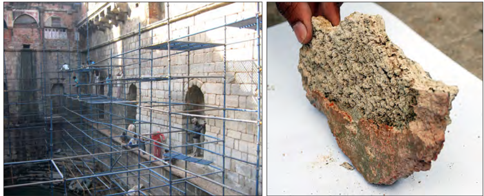
Removing epoxy layer and cement mortar
