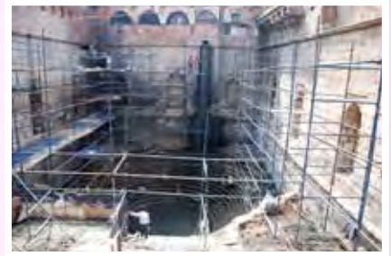
Conservation works in progress
