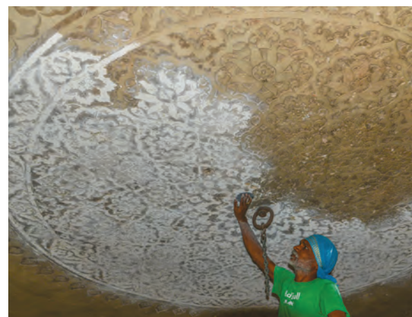
(Top) Mastercraftsman restoring the missing ornamental patterns of the lower arcade in incised lime plaster; (Centre) Craftsmen restoring the lower facade of the tomb; (Bottom) Main Tomb Chamber ceiling during conservation, where the walls and alcoves were cleaned using soft brushes and water.
