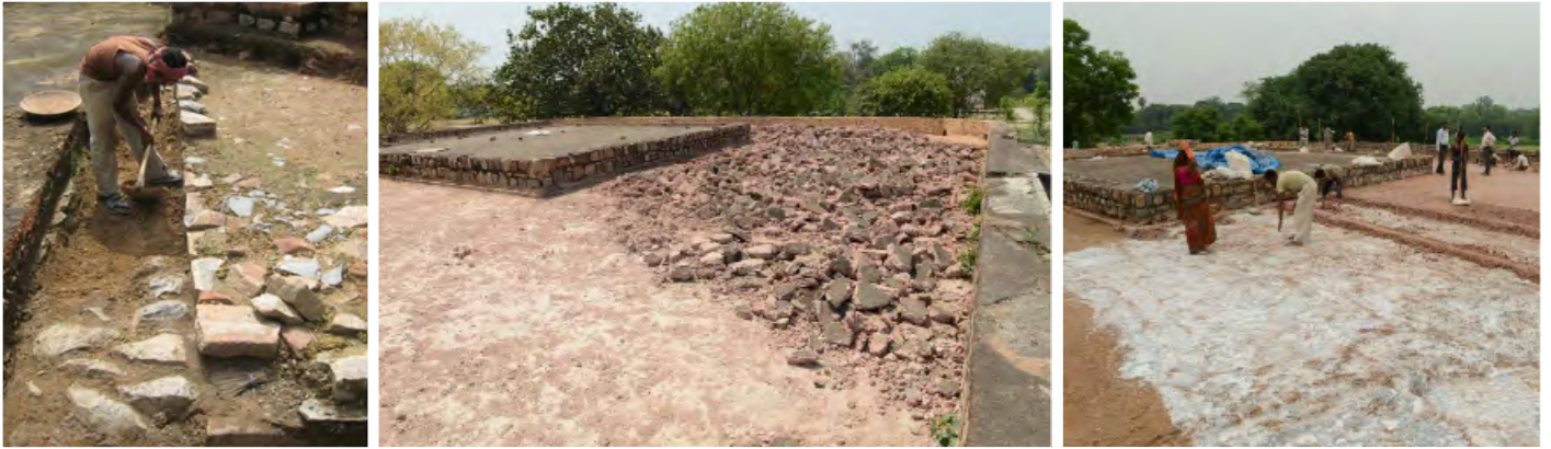
(Left) Dismantling existing cement concrete from flooring; and (Middle) terrace and (Right) laying lime concrete. The final phase of conservation works at Sundarwala Mahal are supported by HUDCO through NCF
